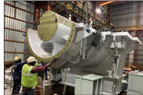
Top Recovery Turbine erection at BF
